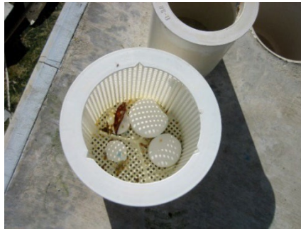
Example of improper dispensing of chlorine in skimmer basket.
