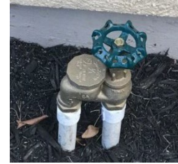
Atmospheric Vacuum Breaker
