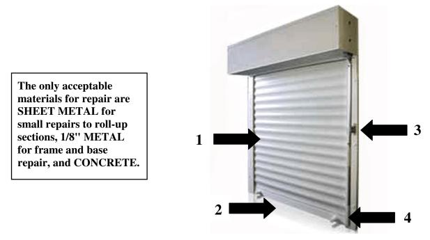
1. Check roll-up sections for damage. Holes larger than 1/4" must be repaired with metal. Roll-up sections with excessive damage should be replaced.
