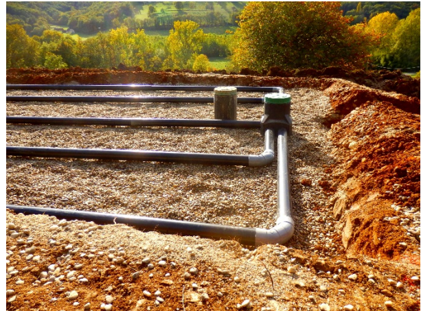
Construction of a Leach Bed
